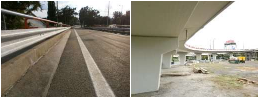
Figure 10. The bridge after the reconstruction works.
