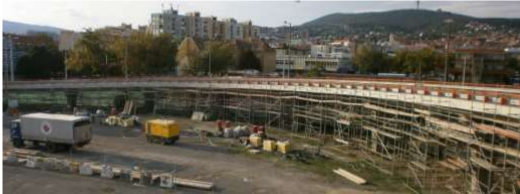
Figure 9. The bridge during the reconstruction works.
